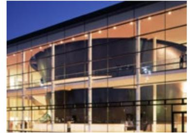
Erfurt theatre: Complete glass facade connected using steel plates integrated into the spun concrete.
