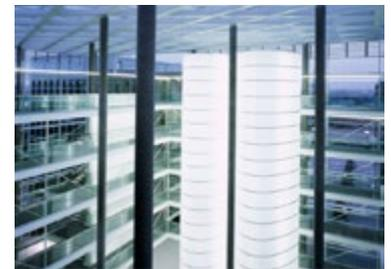
VHV Versicherungen insurance company, Hanover: Columns 25 m long and 0.45 m in diameter
